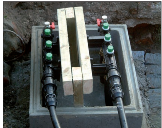
Ground loop pipes
